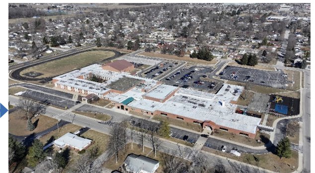
Harris Elementary School (Source: REA)
