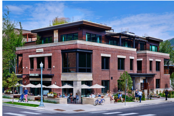
The Spring Building, Aspen, CO (Rudin West Development)
