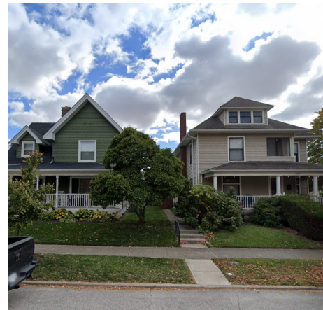
North Street in Greenfield (Google Maps)
