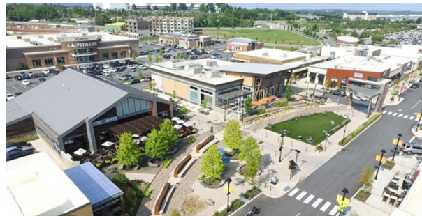
King of Prussia, PA (Source: Citadel Nat. Construction Group)
